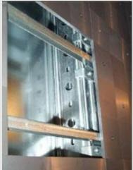
Ferrite panels are screwed onto a metallic sub-structure, made of main and secondary steel profiles. Vertical main profiles are directly fixed onto the shielded room, using the joining OMEGA profiles between two shielding panels. Then horizontal secondary profiles are screwed onto these main profiles.
